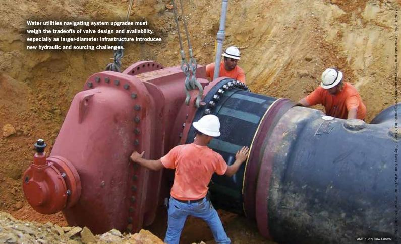
AWWA gate valve standards currently don't exceed the 72-inch nominal size. The use of reducers to accommodate smaller gate valves in a larger pipeline has been a common practice for many years.
