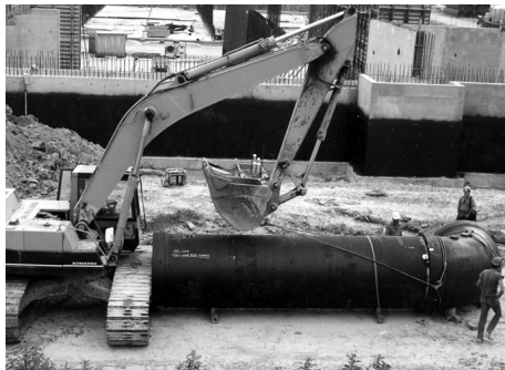
Assembly of a larger push-on joint fitting.
