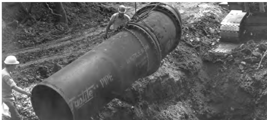
Installing a mechanical joint bend in a gravity sewer utilizing field-cut closure pieces to locate the fitting accurately.
