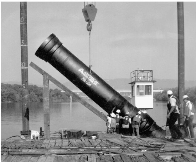
48" Flex-Lok Pipe being positioned for assembly. The ramp attached to the barge is used as the assembly platform, and as the joints are made, the barge is moved forward, allowing assembled piping to slide into the water.
