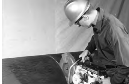
Cutting ductile iron pipe with abrasive wheel.
