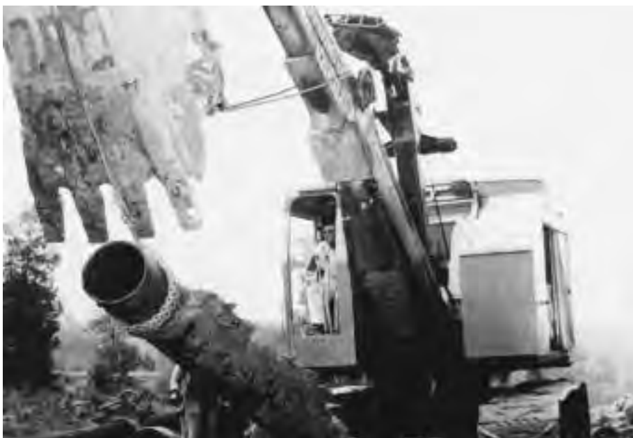
Cast Iron Pipe – being replaced by a larger main – is taken up after years of service for installation in another location for continued service.
