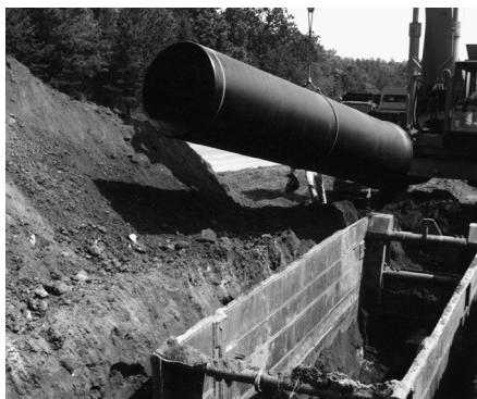
This 30" AMERICAN Ductile Iron Fastite joint treated-water transmission main was furnished and installed—as is most ductile iron pipe—with standard asphaltic coating approximately one mil thick on the outside.
