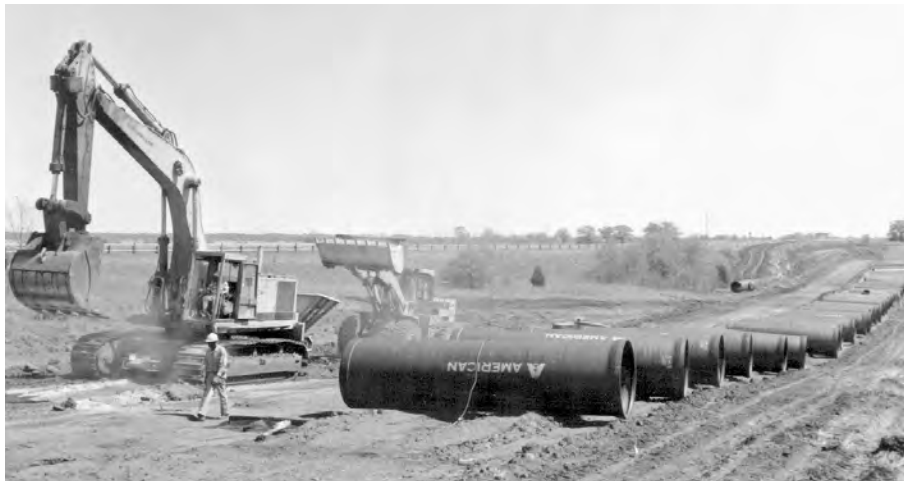
60" AMERICAN Fastite® Joint Ductile Iron pipe being installed as a water transmission main.
