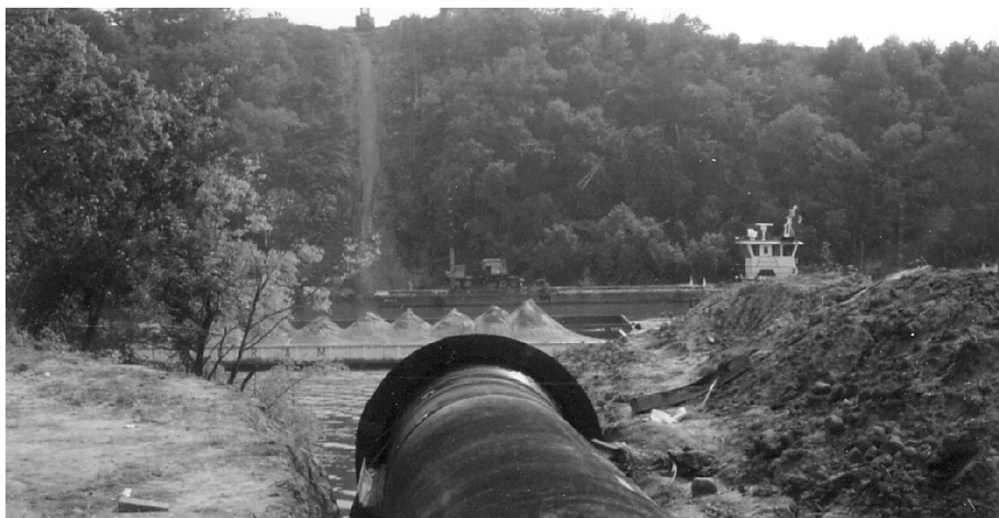
Bank installation in progress, where most of the work is performed on firm ground and the pipe is pulled across waterway by cable. (Note rail weights strapped on to create slight negative buoyancy of this size line pulled beneath barge traffic).
